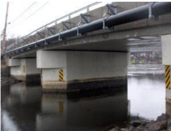
County Bridge #819 – Brady Road Bridge
